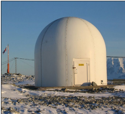
▲ The ARIES Dome captures satellite image data to help with daily weather forecasting
