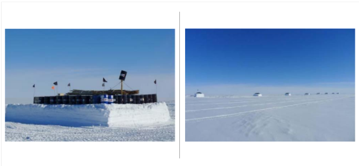
Figure 23. Raised berms used to store fuel (in drums and bladders) during the winter period. Source: BAS Traverse Operations Manual.
