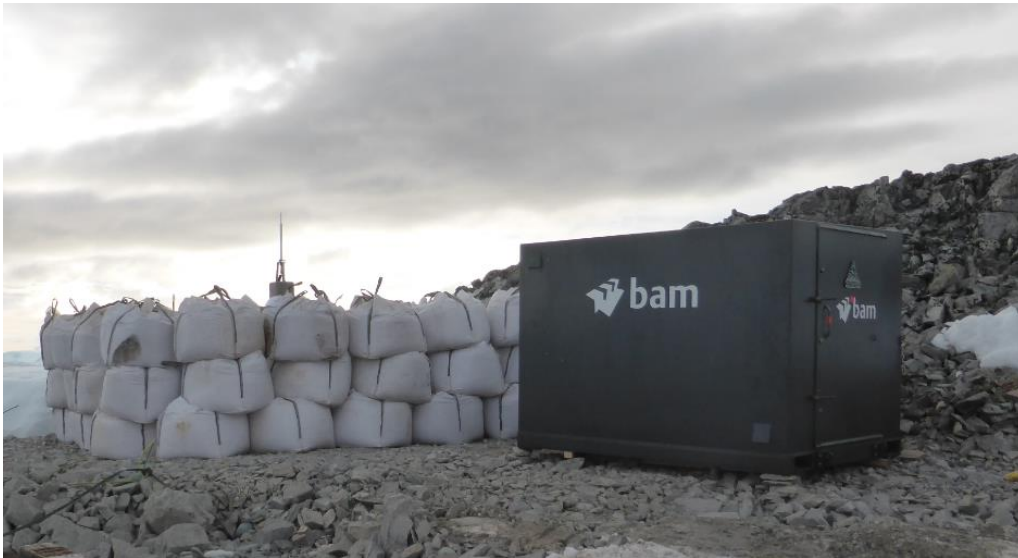
Figure 14 – BAM on-station detonator magazine. The existing BAS magazine is enclosed by the bund.
