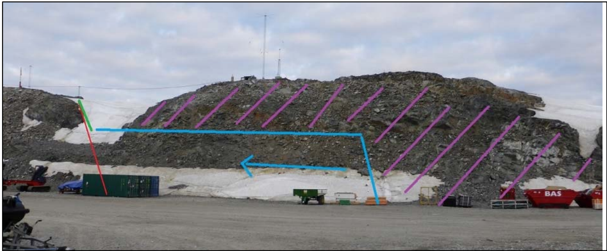
Figure 4-8 Quarry stage 3 showing the upper bench worked out, production continuing on the lower bench.
