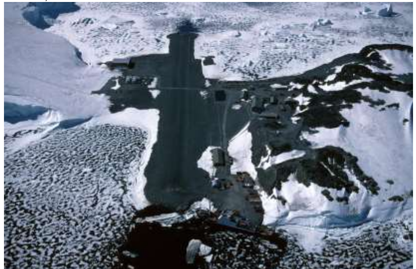
Phase I, a small accommodation block was
