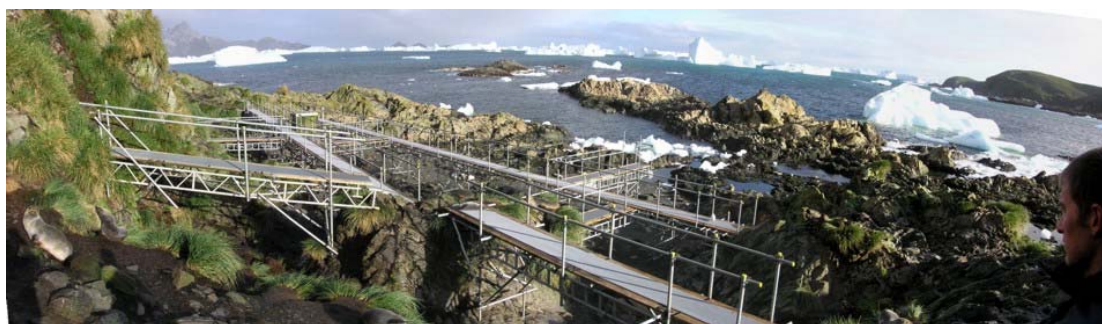
AFTER: The Seal Study Beach with the new scaffold walkway
