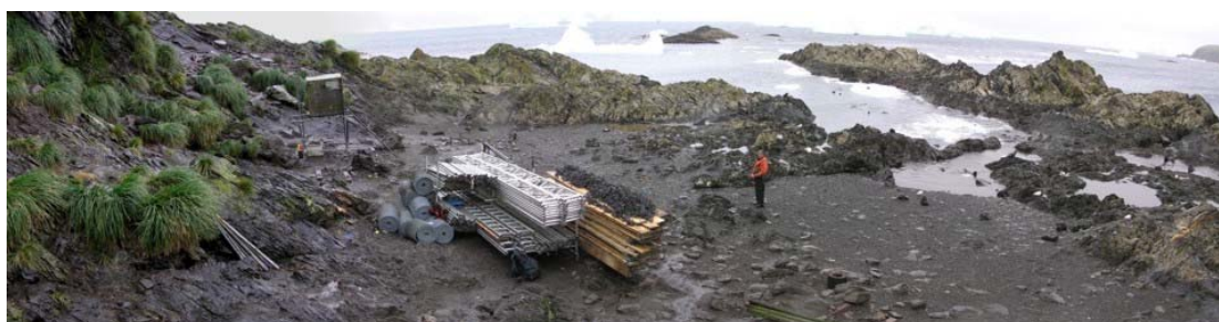
BEFORE: The Seal Study Beach with the old scaffolding removed
